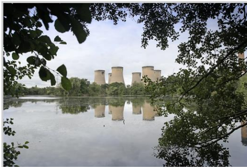
Drax Power Station
