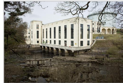
Tongland Power Station
